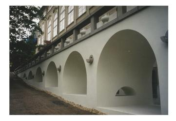
The contracting company responsible for the work was ABV s.r.o. Praha 9. Xypex Concentrate, Xypex Modified, and Xypex Patch'n Plug were selected to waterproof the ancient masonry. These Xypex products provided the project with a permanent waterproofing solution, playing a crucial role in enhancing the waterproofing capabilities of the bridge and contributing to its preservation and longevity amidst its high-profile location.
